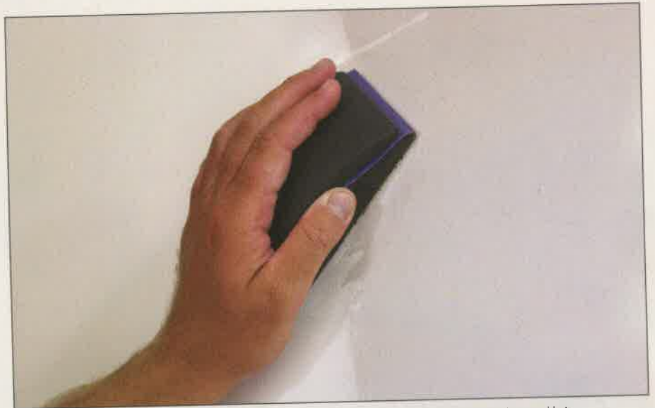
Rigidity is the key to skiving off bumps and imperfections. A rubber sanding block fitted with sandpaper is a good bet.
